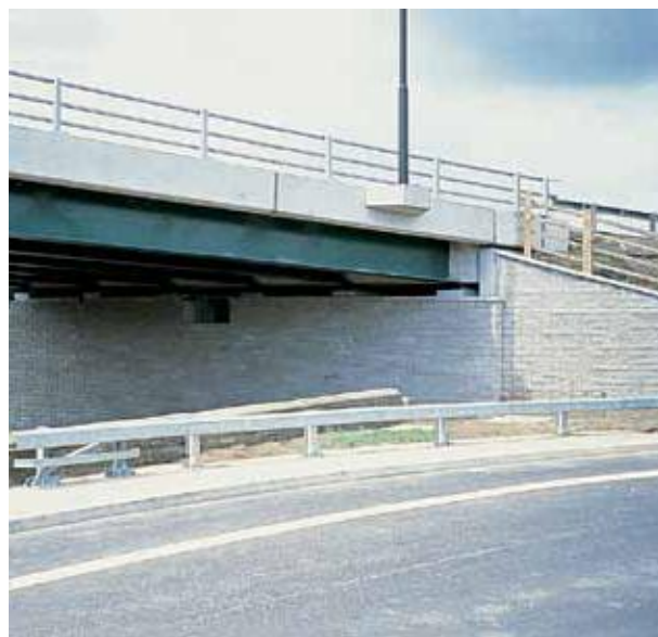
TensarTech Systems have been independently certified for use as load bearing bridge abutments in highway applications by the British Board of Agrément.
