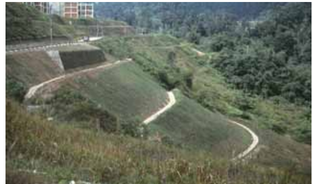
Appropriate face detailing allows vegetation to quickly establish.
